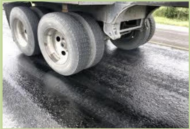
**CleanTac** is an anionic setting asphalt emulsion with superior bond strength designed for use as a Fast-drying tack coat, in finegraded mixes, and specialty applications to help eliminate tire tracking. It is formulated with a harder base than SS-1 for use in warmer climates. Designed to hold asphalt layers together with the new and old surfaces, but not to tires and equipment, CLEAN TAC keeps cleanup to a minimum at a lower cost.
